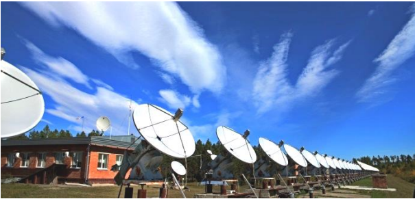
Figure 2. Part of the antenna array SRH-48. Antenna diameter is 1.8 m; distance between antennas is 4.9 m. The larger remote white antennas belong to the SSRT array. Signals from the SRH antennas are transmitted via fiber links in the tunnel to the working building visible behind the antennas
